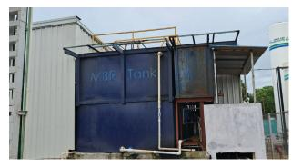
Once treated, the water is seamlessly integrated back into our operations for various processes, including cooling towers, chiller units, and forming machine cooling, effectively closing the loop on water consumption. With a robust capacity of 120 kiloliters per day (KLD), our ZLD system exemplifies our unwavering commitment to environmental stewardship.
