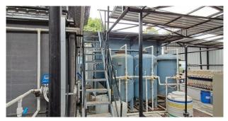
The effluent then undergoes tertiary treatment stages, including dual media filtration, & activated carbon filtration (ACF), ensuring the highest level of purification. Subsequently, the treated water undergoes additional polishing through ultrafiltration and reverse osmosis (RO) at three stages to meet stringent quality standards.
